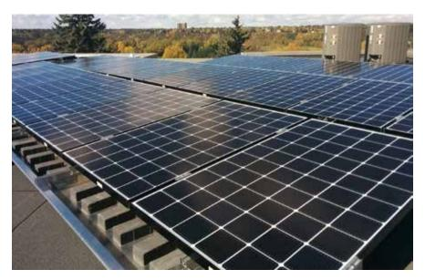
The building will have solar photovoltaic (PV) arrays on all available roof areas to produce as much renewable energy as possible, offsetting the building's overall energy reliance on the grid and reducing the project's annual operational costs.
